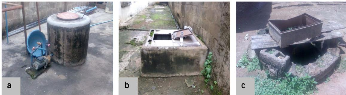
Figure 2: Construction patterns of selected wells - a: protected well; b: semi-protected; c: unprotected well
